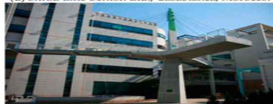
(f) The world's first UHPC pedestrian cable-stayed bridge.
